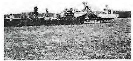
Traditional wheel trenching drainage machine laying clay tile.
