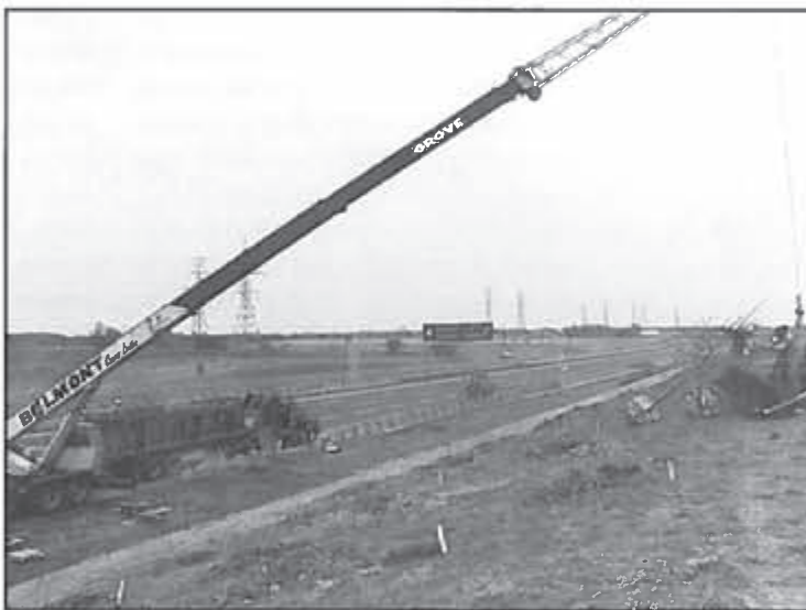
A large crane greatly facilitated the job of planting caliper trees on the steeply sloped roadsides of the newly constructed Highway 403.
