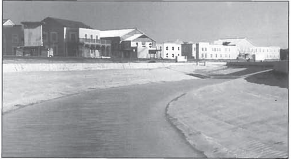
A Carlisle EPDM pond liner was used to line a 1.2 million sq. ft. man-made lake at EURO-DISNEY near Paris, France.
