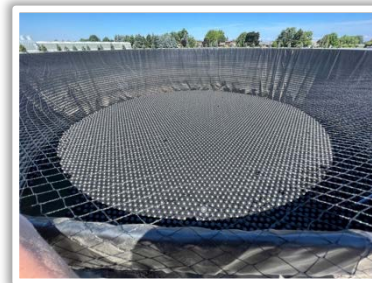
Bird Balls covering a silo surface.
