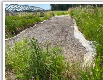
A hybrid treatment swale at a container nursery.
